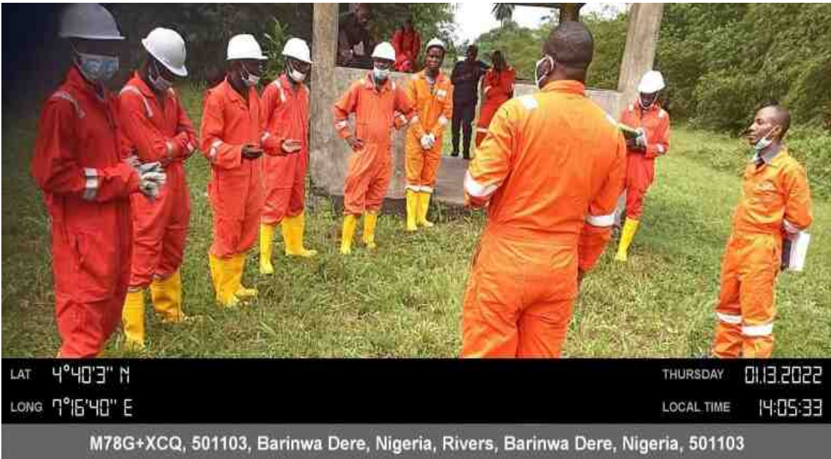
Induction Along 28" Nkpoku-Bomu Pipeline At B.Dere
