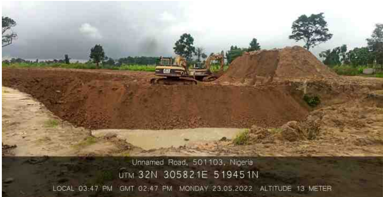
Backfilling of Section A and B with treated soil
