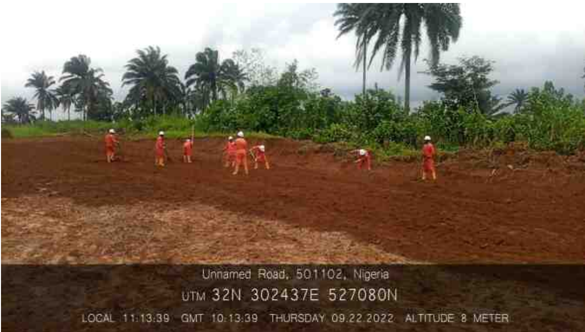
Manual breaking of windrow
