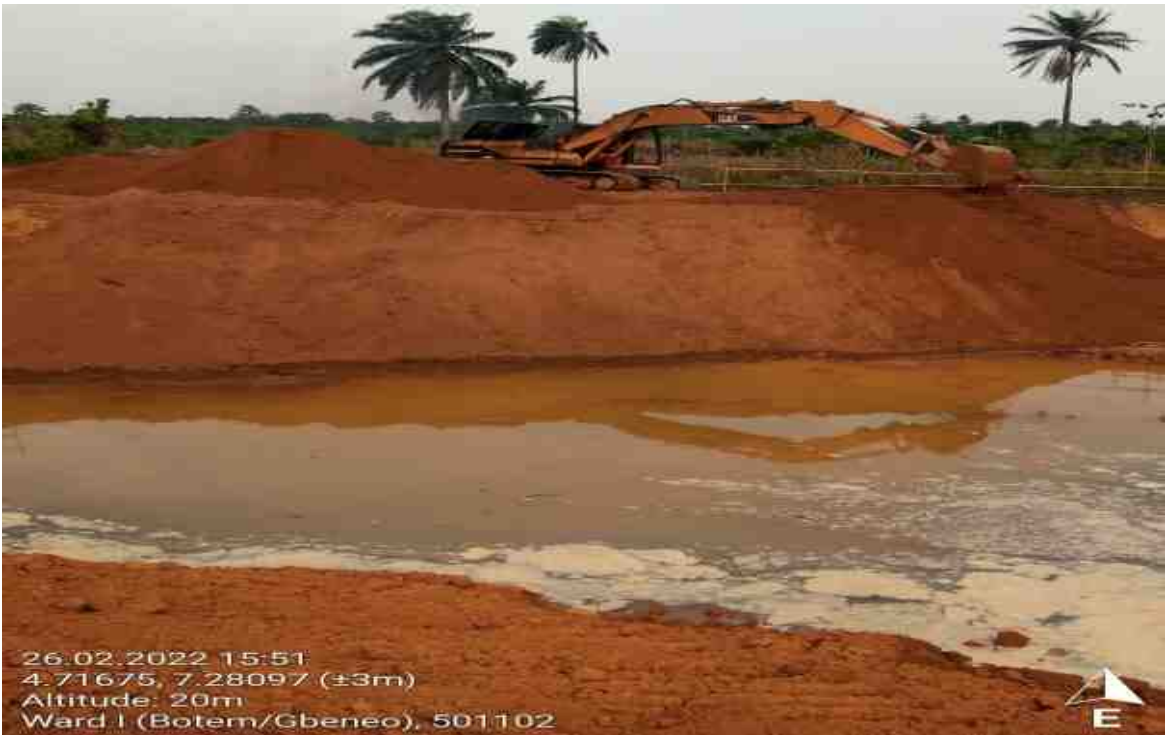
Backfilling of excavated area
