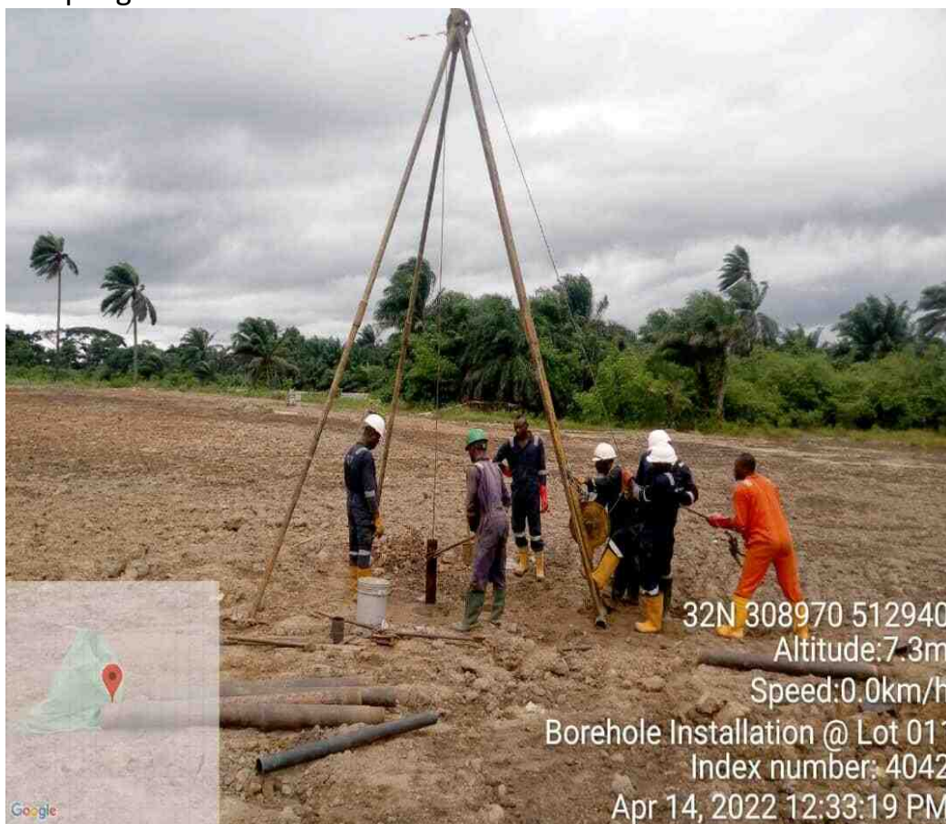
Installation of monitoring boreholes at the completion of remediation
