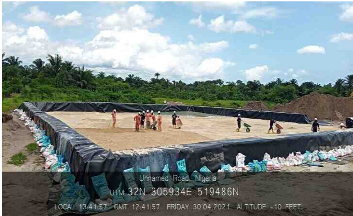
Leveling the Biocell with 0.2m sharp sand layer for leachate permeability
