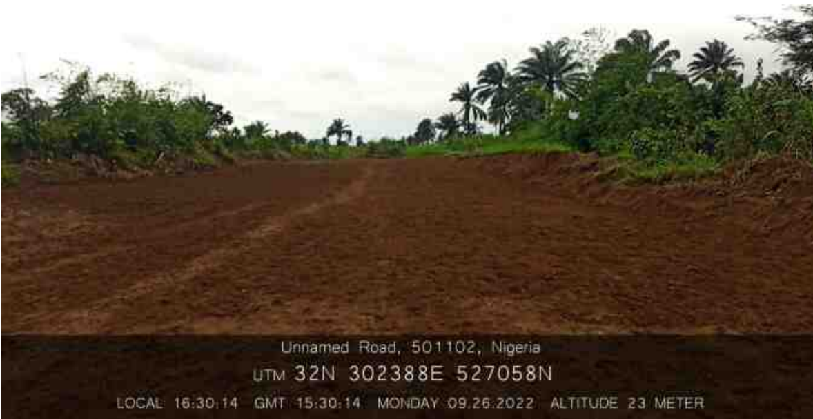
Site after remediation
