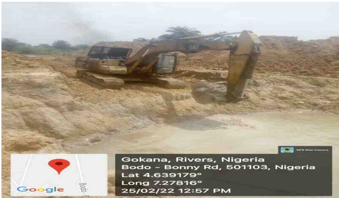
Excavation of impacted area
