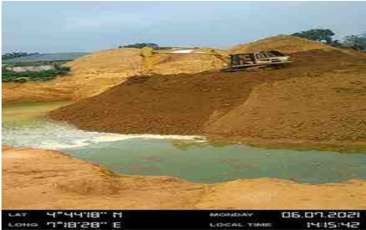
Backfilling of Excavated area
