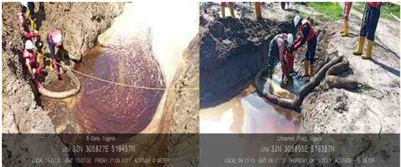
Recovery of Free phase crude oil from excavated trench
