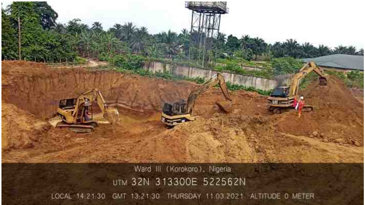
Excavation of Impacted area
