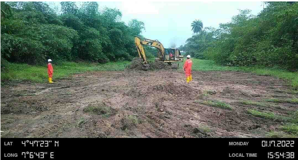
Mechanical clearing of impacted area
