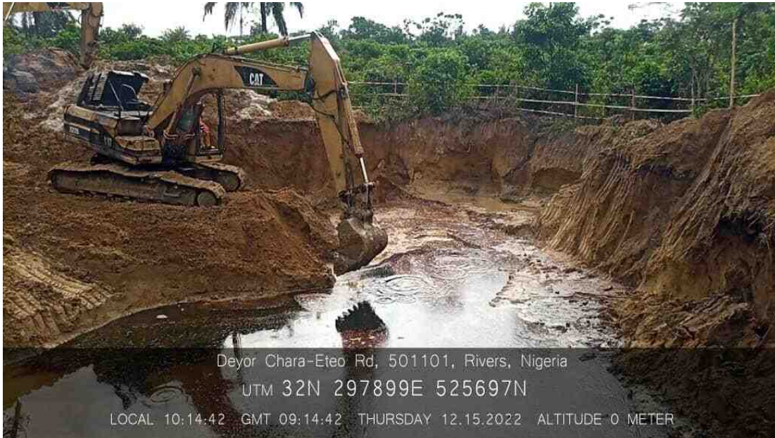
Deep Excavation at the depth of 5m
