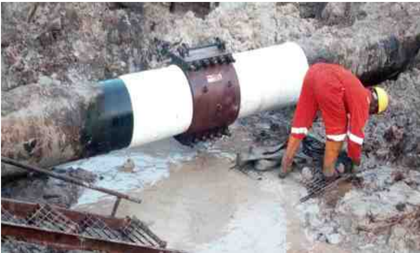
Clamping Of 24'' at Biara Site in Ogoni
