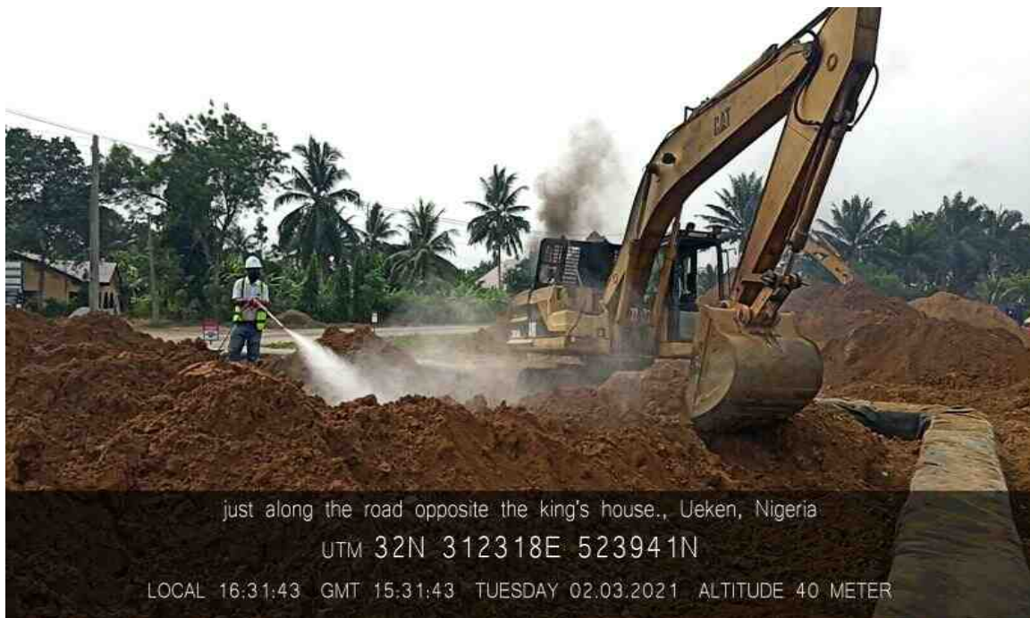
Treatment and homogenization of impacted soil
