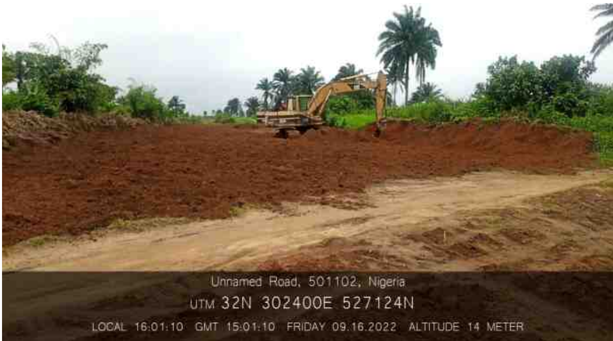
Tilling and homogenization of impacted soil in section B
