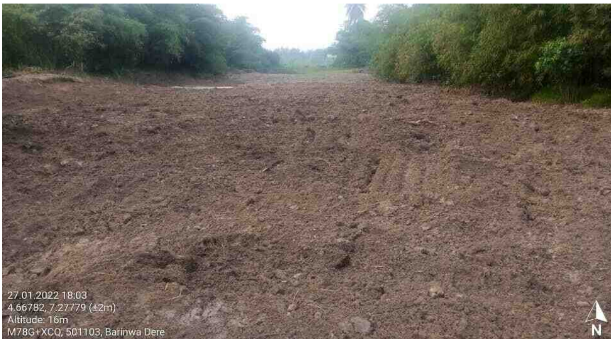
Completion Back Filling OF Trenches
