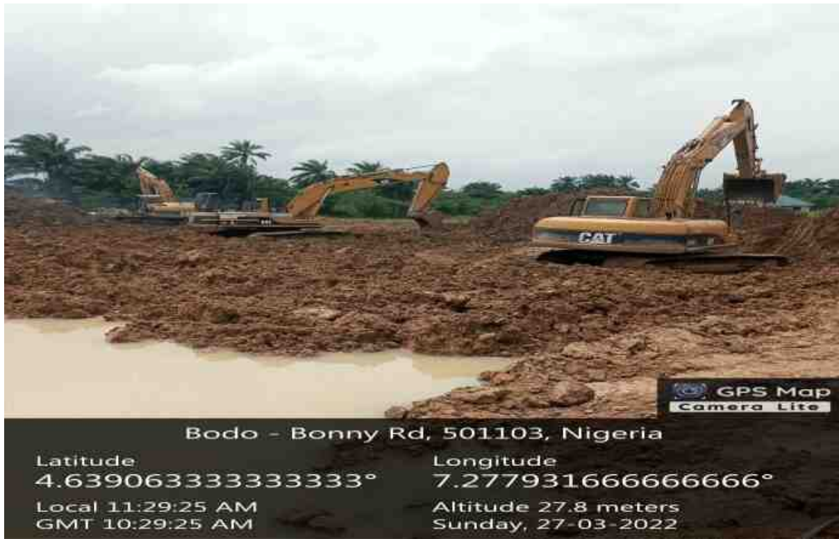
Backfilling of treated soil
