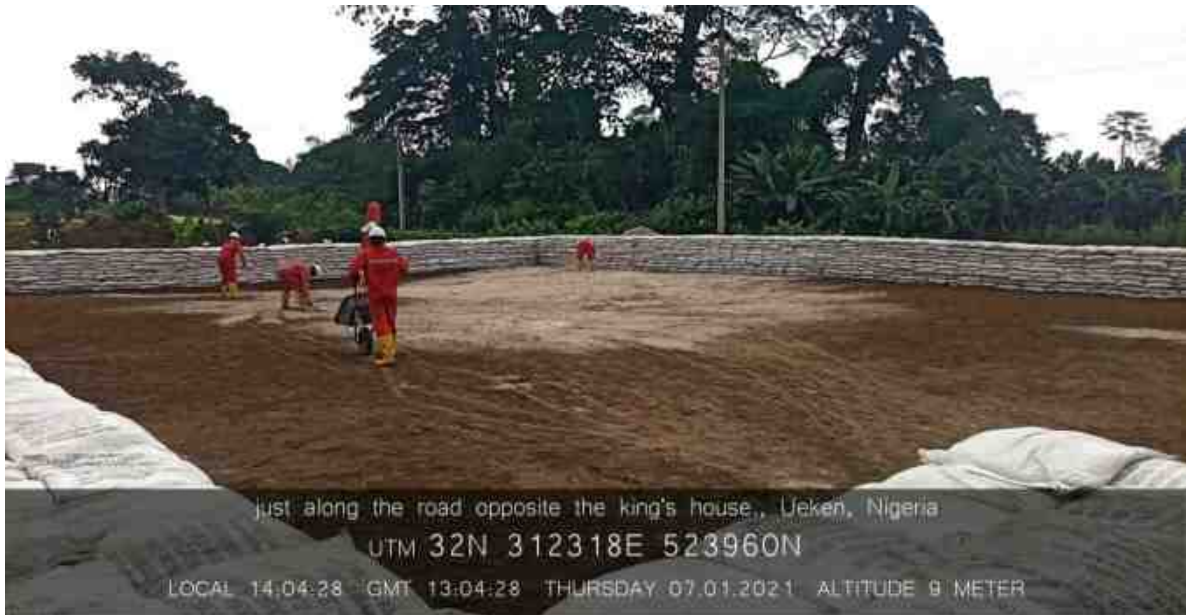
Engineered Biocell Construction
