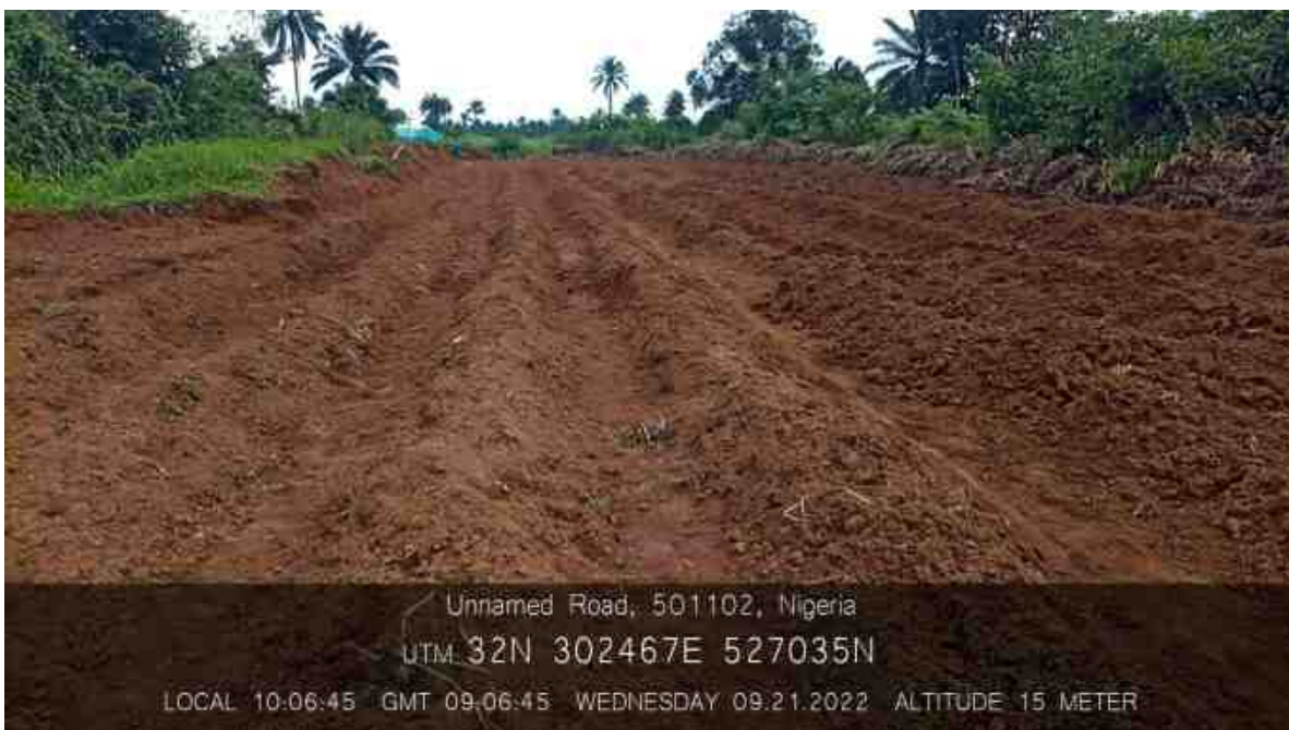
Construction of windrows in section B
