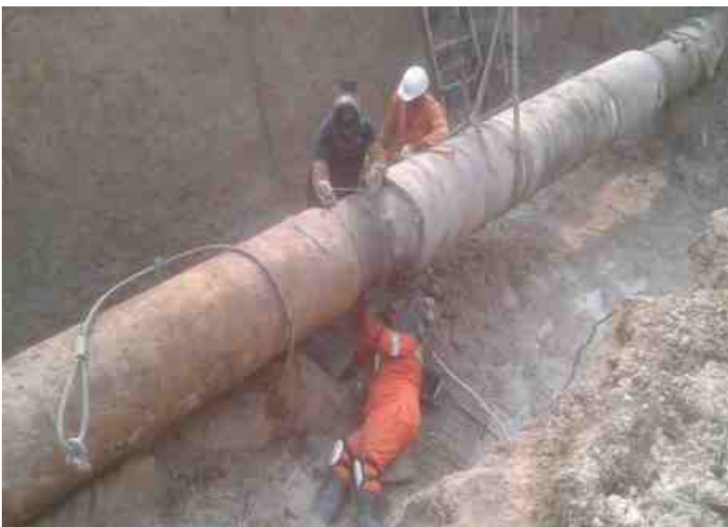
Sectional Replacement 24'' at Sime, Tai
