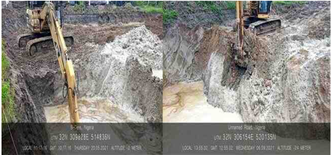
Deep excavation of impacted soil
