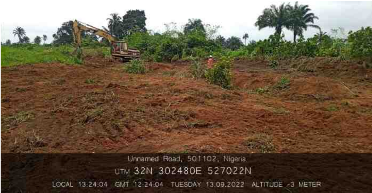
Clearing of delineated impacted area for remediation
