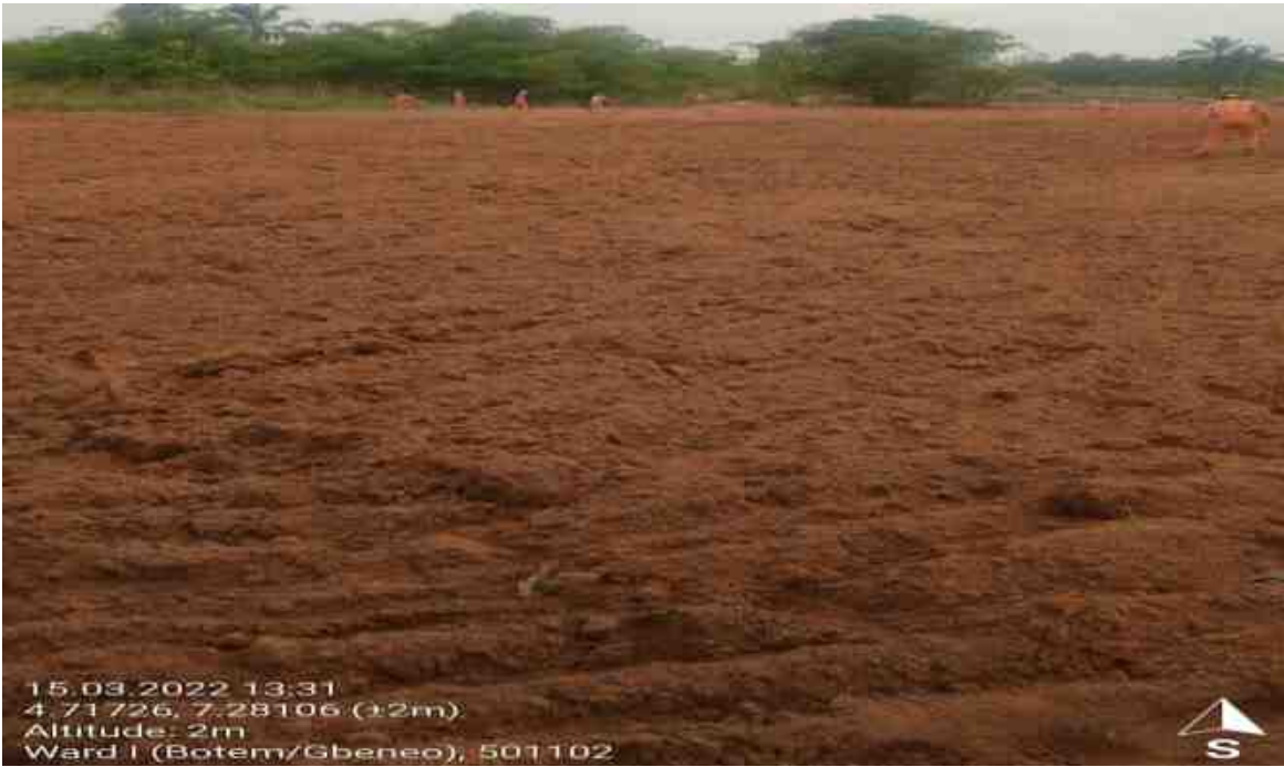
Landscaping of excavated site
