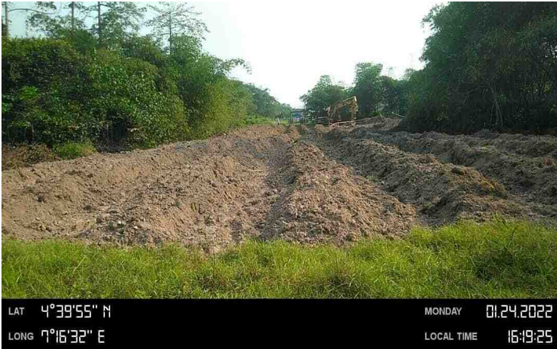
Constructed of Windrows and treatment of impacted soil
