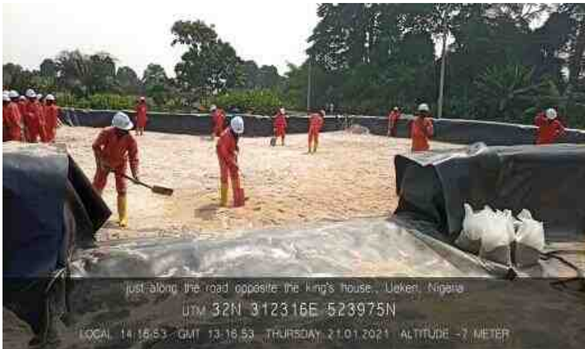
Constructed Engineered Biocell
