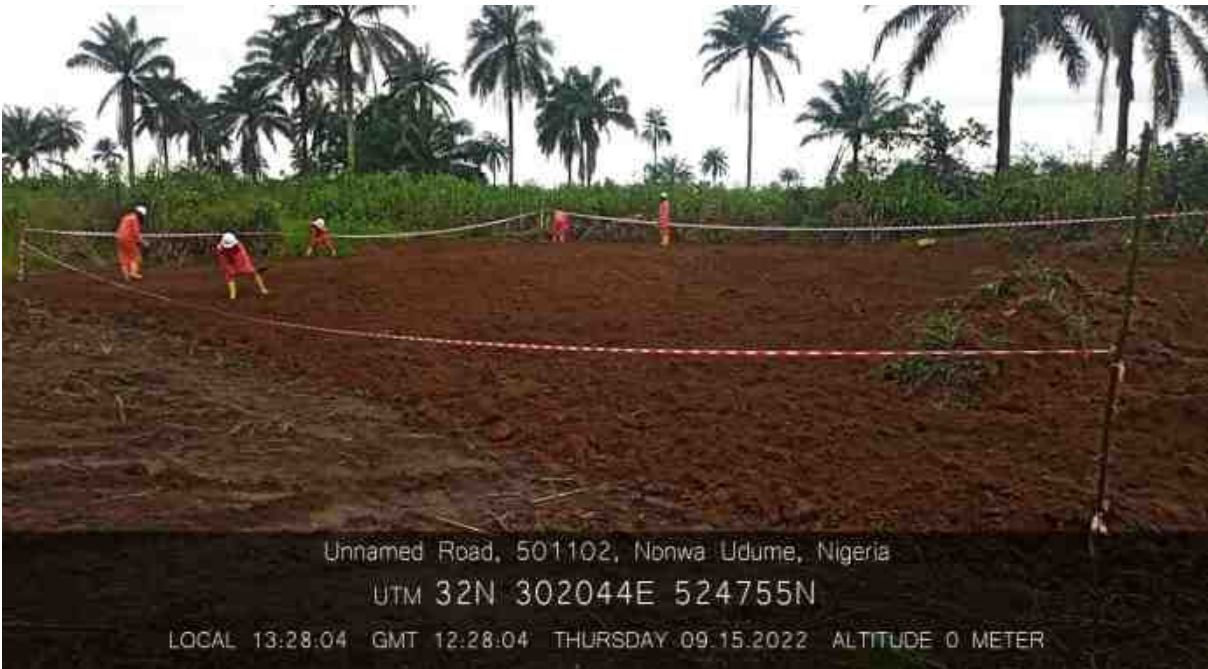
Tilling, homogenization and manual breaking of soil lumps in section A
