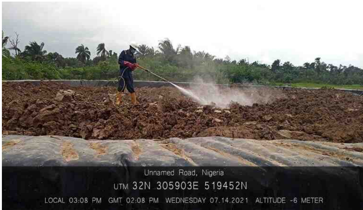
Treatment of impacted soil
