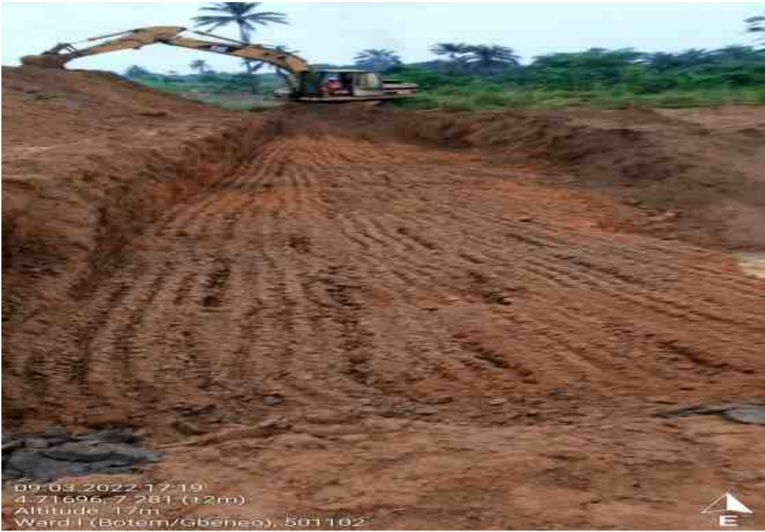
Excavation of Extension Area
