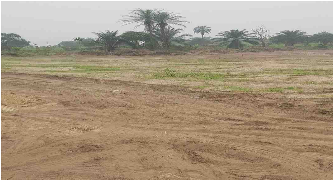
Site Clearing and grading
