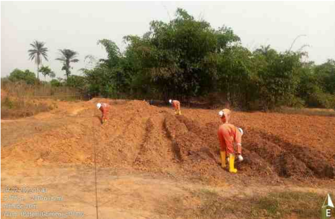
Construction of Windrows
