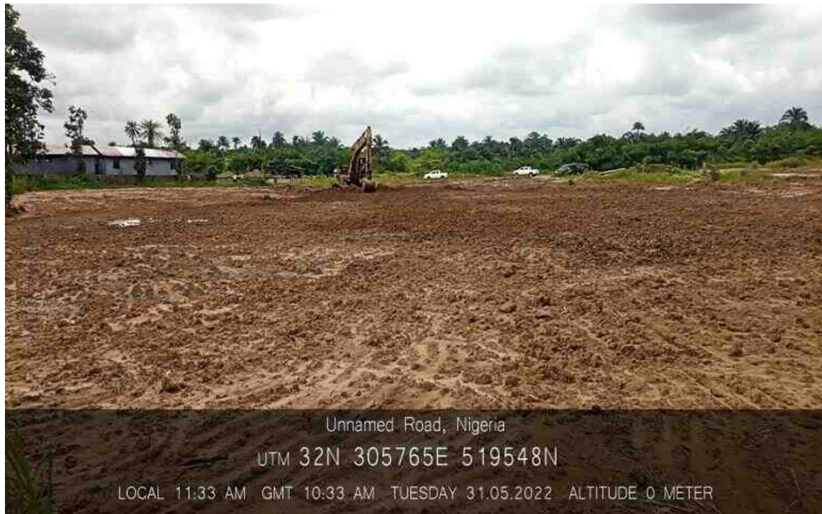
Landscaping of Backfilled area
